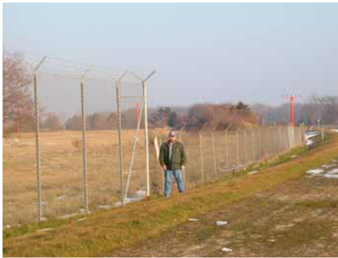
A well-maintained fence, at least 10-feet high with no gaps at the bottom, is the primary defense to keep deer and other large animals off the airport's AOA. Deer can easily jump fences that are only 6 feet high (right) (photo by R. A. Dolbeer, USDA).
